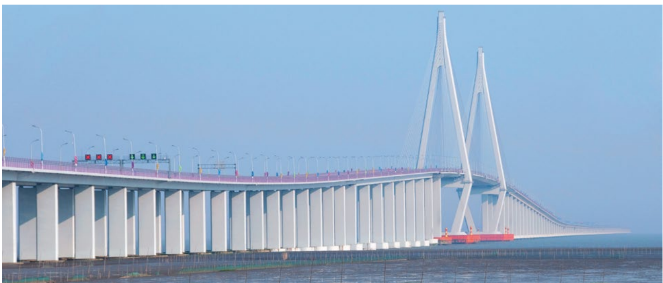
The 7,000 piers of the Hangzhou Bay Bridge in China are anchored in the seabed. Protectosil® CIT protects them against penetration of water and chemicals
