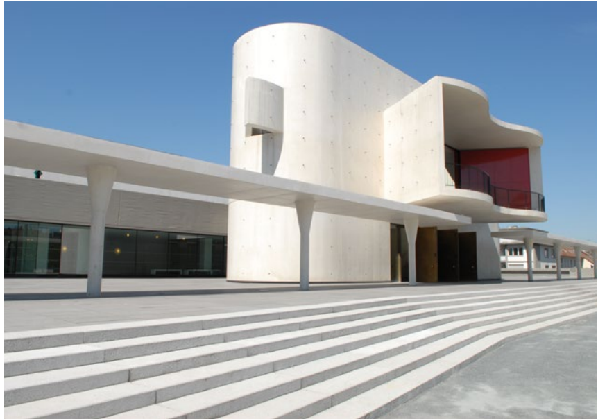
Protectosil ANTIGRAFFITI® protects the white marble facade of the State Theatre in Darmstadt, Germany
