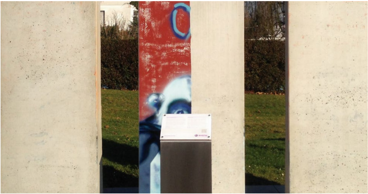
Concrete wall after removal of graffiti
