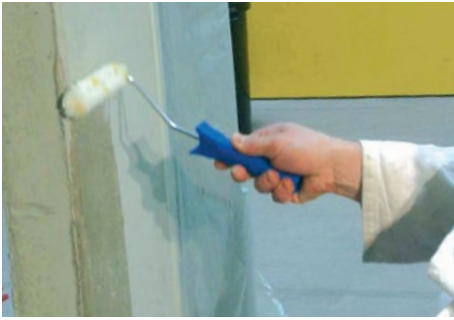
Application of Protectosil ANTIGRAFFITI® SP
