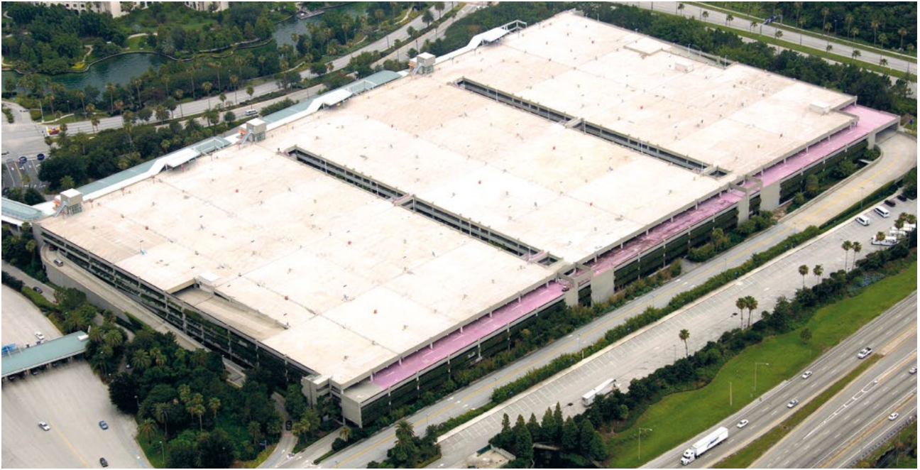
The parking areas of Universal Studios in Orlando, Florida, USA have been protected against corrosion by Protectosil® CIT
