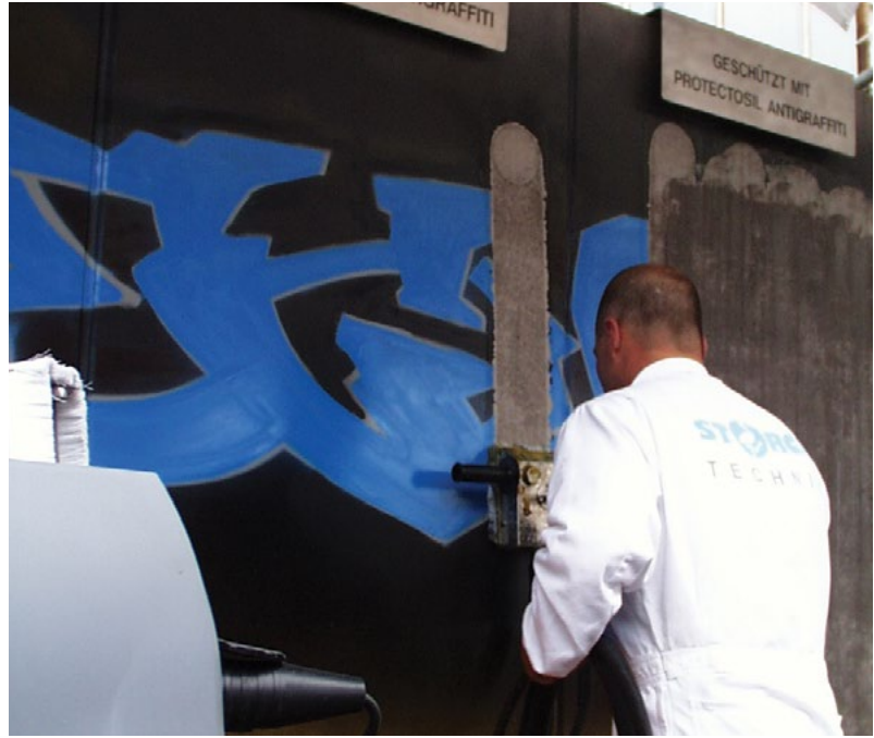
Cleaning of a wall with graffiti art
