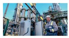
A new sampling station at the oxo plant in Marl (Germany) automatically takes daily samples of wastewater for analysis.
